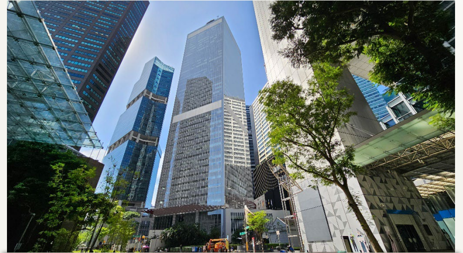
Works are in progress for the asset enhancement of the Singapore Land Tower (centre).
